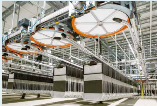
Vanderlande's hanging high-speed sorting system
